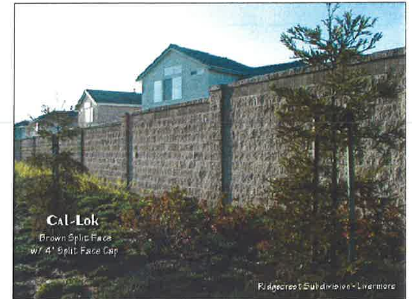
Typical Perimeter Wall ("CAL-LOK WALL SYSTEM")
